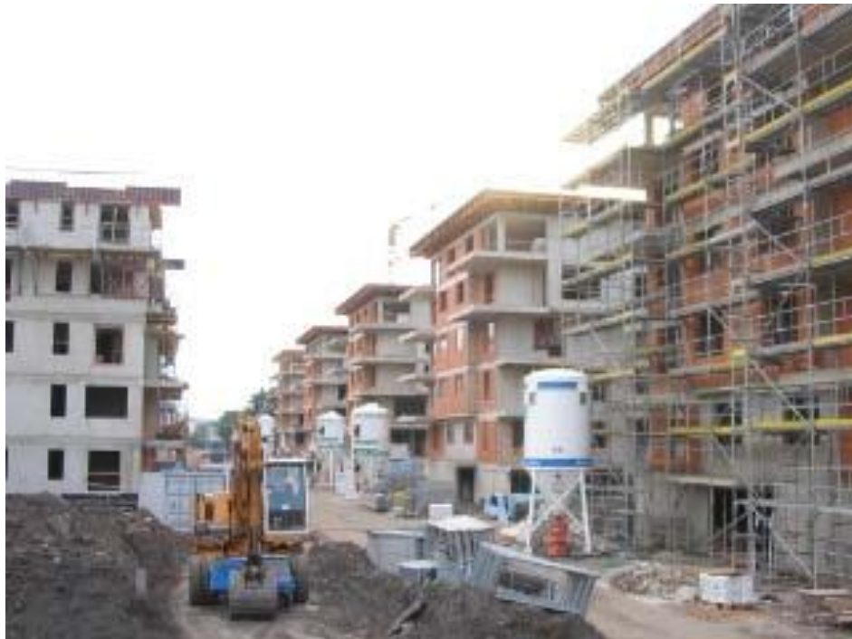
Photo 6 - Courtyard Building Underway
